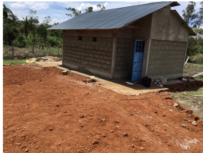
Restrooms and showers for the Bible college in Kenya
