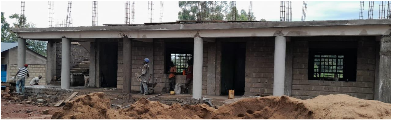
Dorm construction for the Bible College
